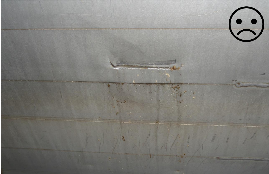
Figur 12. Skade/revne i vognside – AFVIST / Damage/crack in side of truck – REJECTED.
