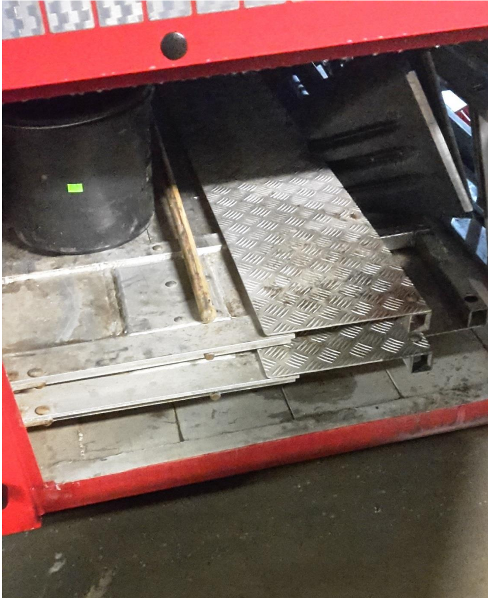
Figur 21. Magasinrum med ekstra stiskillerum. Skal ud og efterses / Compartment room with an extra path partition compartment. This has to be taken out and inspected.
