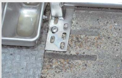
*Corrosion of slatted floor in a pen floor treated with an impregnation product.*
