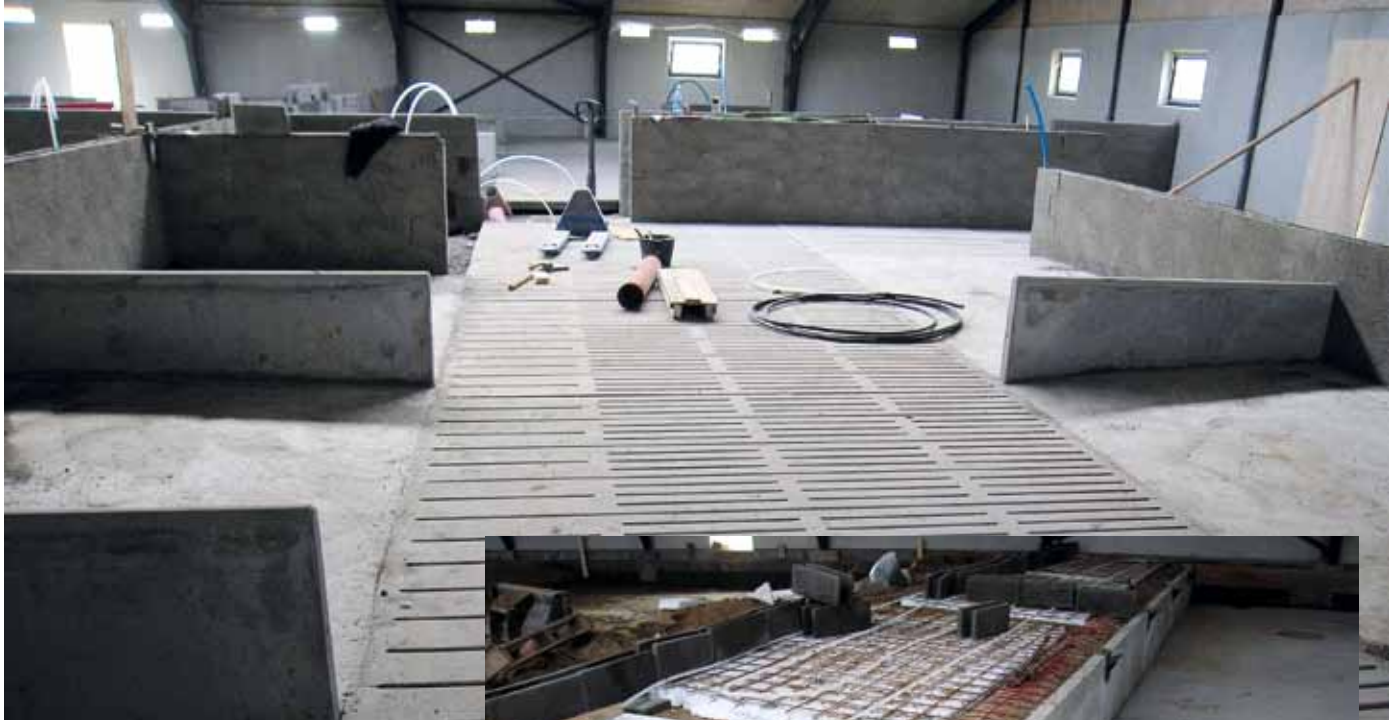
Installation of nozzles and cross-over flue in a gestation house with electronic sow feeding. The channel for point extraction is placed just below the solid floor by the transition to the slurry pit.
