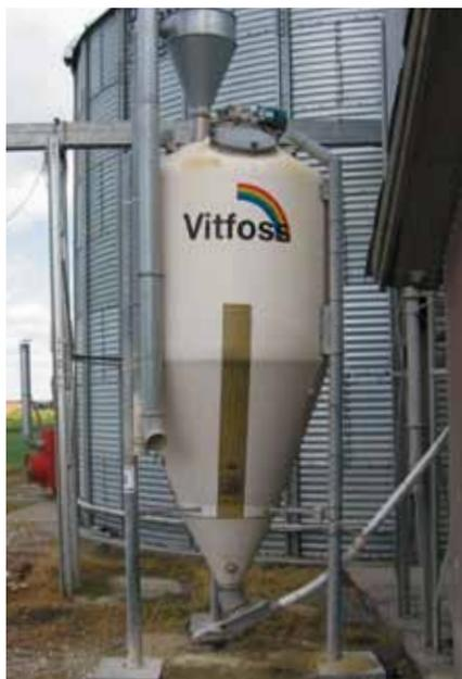
*Segregation was observed in big bags and in polyester silos, whereas no segregation was observed in fibreglass silos.*
