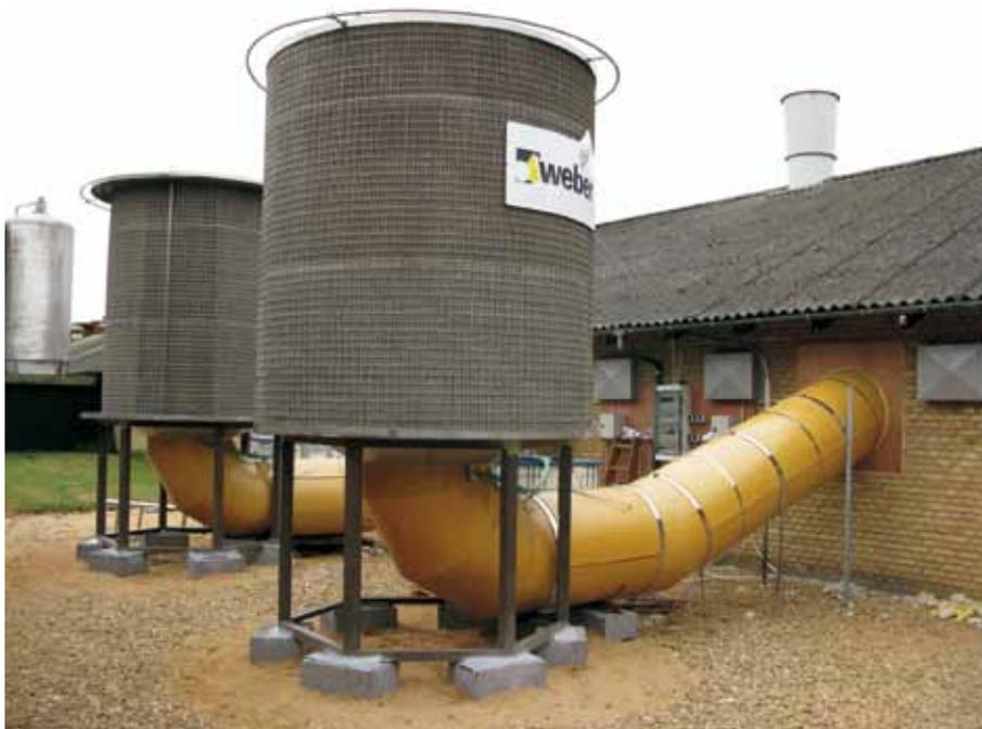
Together with Saint-Gobain Weber, two air cleaning modules with LECA® as filter material are set up in a finisher section at Experimental Station Grønhøj. Reductions in odour and ammonia emissions in the trial modules will be recorded in 2011.
