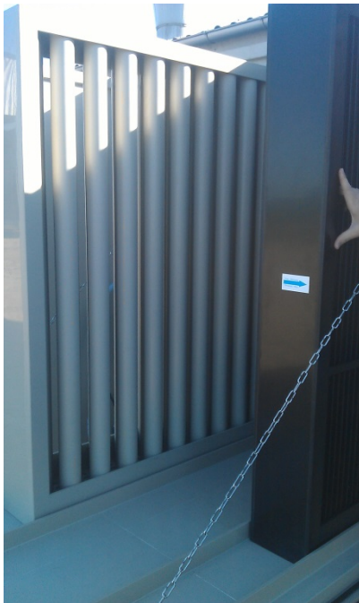
Figure 2. The two mist eliminators can be slid out manually when cleaning the system.
