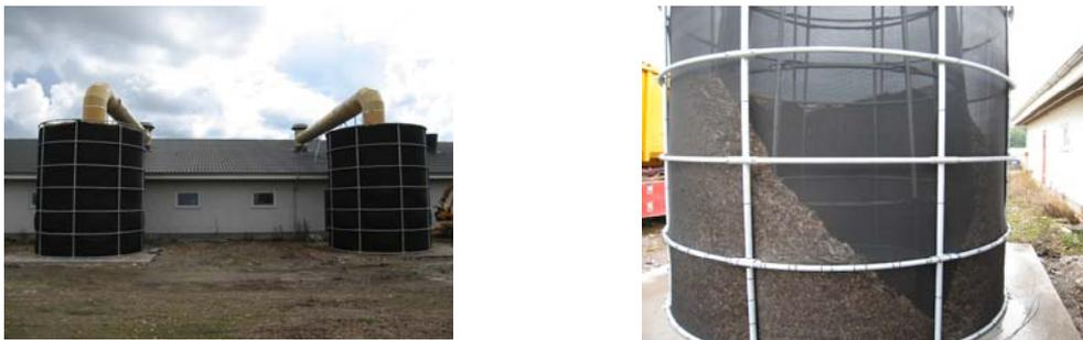
Figure 1. Design of the vertical biofilters.
