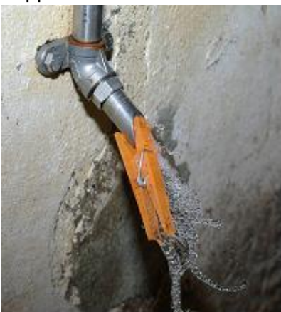
A simple method for flushing of pipes
