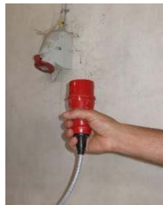
Pull the plug when cleaning the unit. All units must have a plug.
