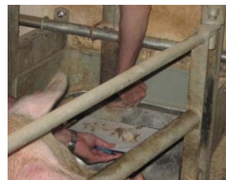
Regularly check for dirt and grease in pipelines between feeders and troughs in the sow facility as this may lead to sudden deaths and reduced milk yield
