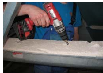
Akku-drill dismantles plate above U-channel
