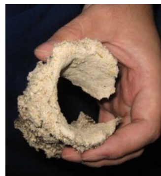
Dirt and grease in pipelines can be removed by brushing or washing
