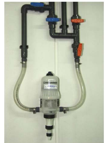
Medicator is connected to the section/pen housing pigs to be treated
