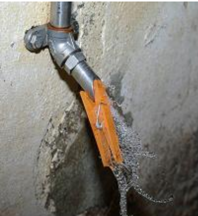
A simple method for flushing of pipes
