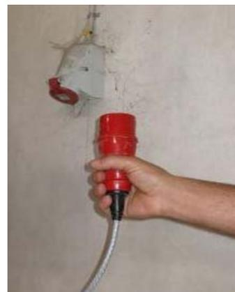
Pull the plug when cleaning the unit. All units must have a plug.
