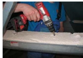
Akku-drill dismantles plate above U-channel
